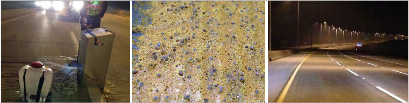
Figure 3.3 Taking a retroreflectivity (continuous wetting, left) reading on I-355 along with marking presence images for the yellow edge line (center) and general photo of all lines (right).
