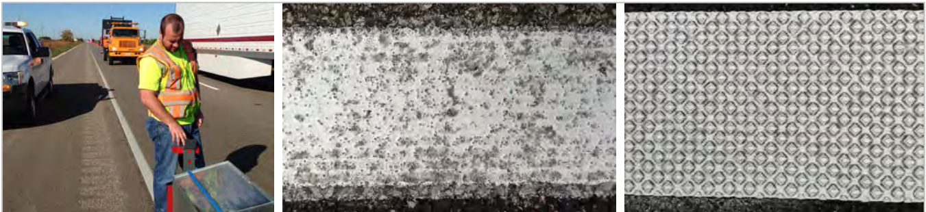
Figure 3.1 Taking a retroreflectivity (continuous wetting, left) reading on I-80 along with marking presence images for the white edge line (center) and centerline skip (right).
