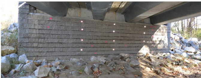
View of Rustic Road GTRS-IBS north abutment with reflective survey markers
