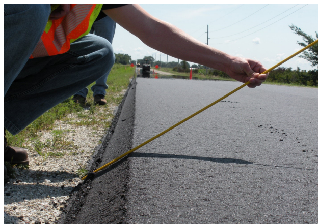
A 30-degree slope on a safety edge.
