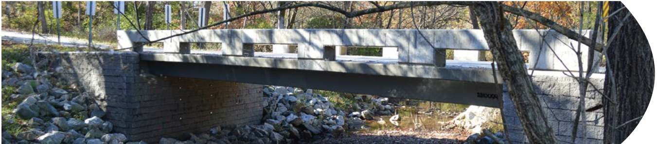
Completed rustic road Geosynthetic Reinforced Soil-Integrated Bridge System from a past research project highlighted below
