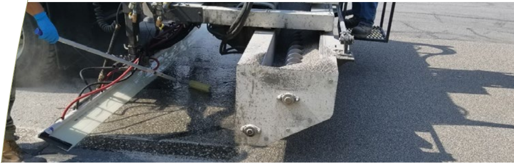
Example of high friction surface treatment application
